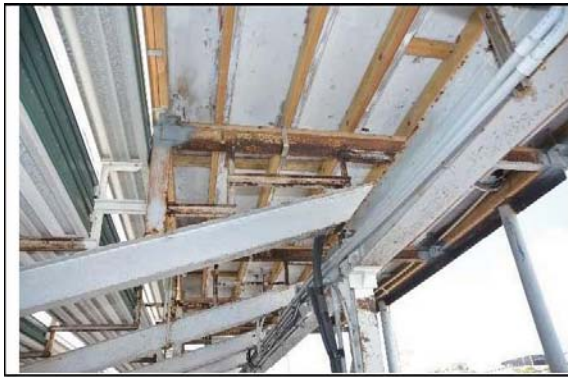
Corrosion of HSS at press box
