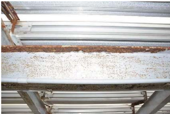
Typical corrosion at connections Corrosion at connections
