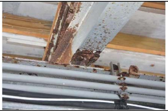
Corrosion of I-beams at press box
