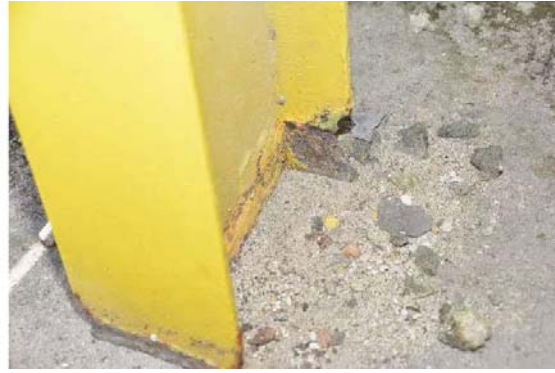
Corrosion at horizontal seat support Corrosion/Spalling at column base
