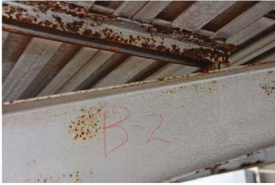
Corrosion at horizontal seat support Corrosion/Spalling at column base
