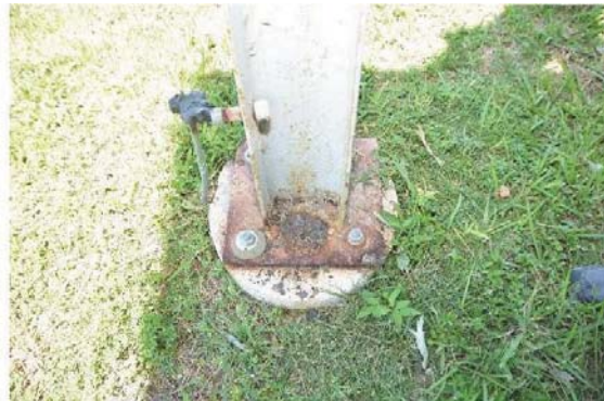
Typical corrosion at connections Corrosion at connections
